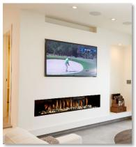
• **Reveal:** A reveal is a popular choice for a heat release design. It allows for the cleanest and most unobstructive aesthetic. A gap is left between the entire chase and the room ceiling, creating a shadow-line effect.
