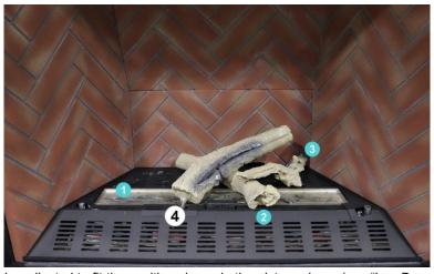
The base/tube for log #4 can be adjusted to fit the position shown in the picture above (see "Log Base Position Adjustment" section for details).
